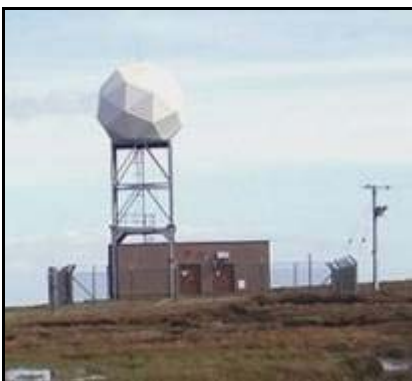
Figure 6. Weather radar, Stornoway, Isle of Lewis.
