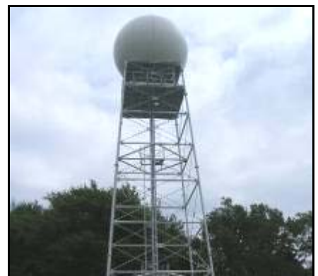
Figure 8. Weather radar, Dean Hill, Wiltshire.
